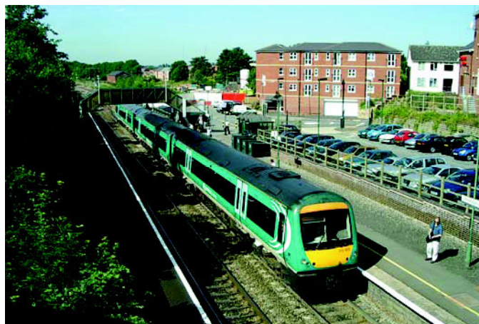
Figure 34: Bromsgrove Train Station
